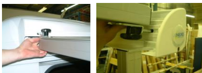
Fig 5. Insert the side rafters
