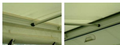
Fig 7. Insert the centre rafter
